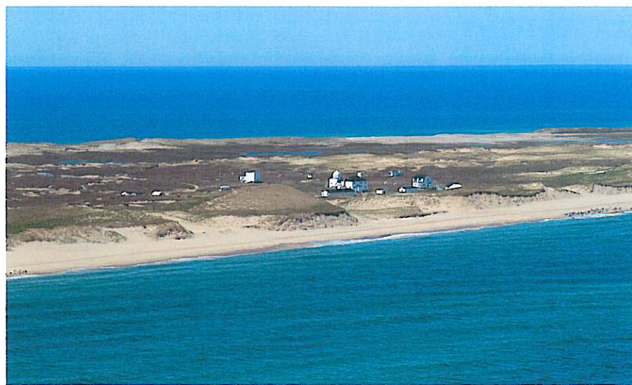
Figure 7 – Aerial View of Sable Island Facilities
