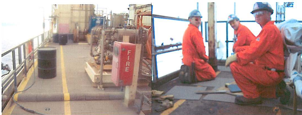
Figure 1 – Local Tradesmen working on Thebaud Deck Restorations
