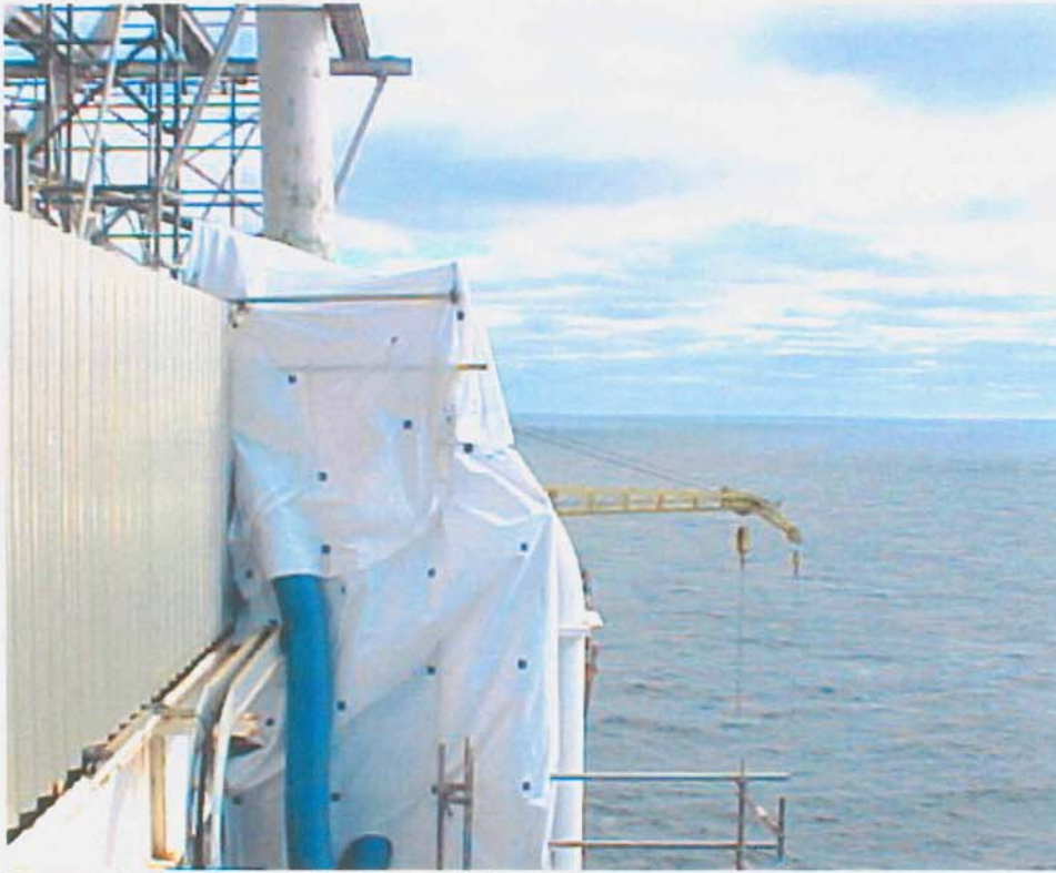
Figure 8 - Offshore Welding Habitat
