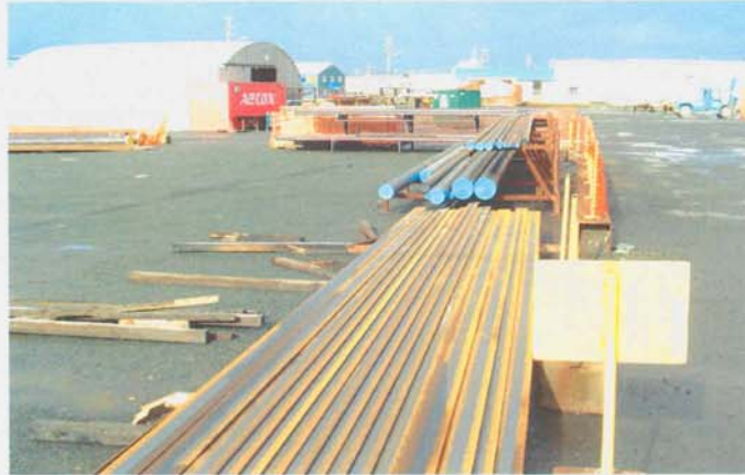
Figure 17 – Beams and Pipes for fabrication of South and East Pipe Racks at Aecon-Fabco, Dartmouth (for Brownfield Modifications - WP03)
