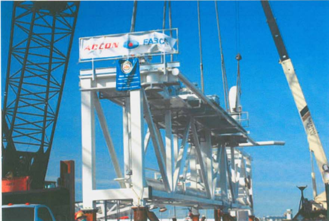
Figure 4 - Pipe Rack at Aecon-Fabco
