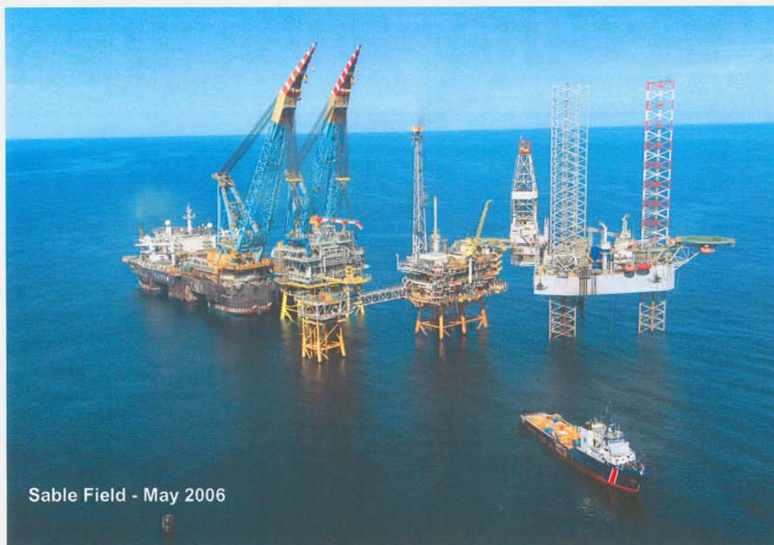
Figure 9 - Saipem SSCV S7000 lifting compression deck
