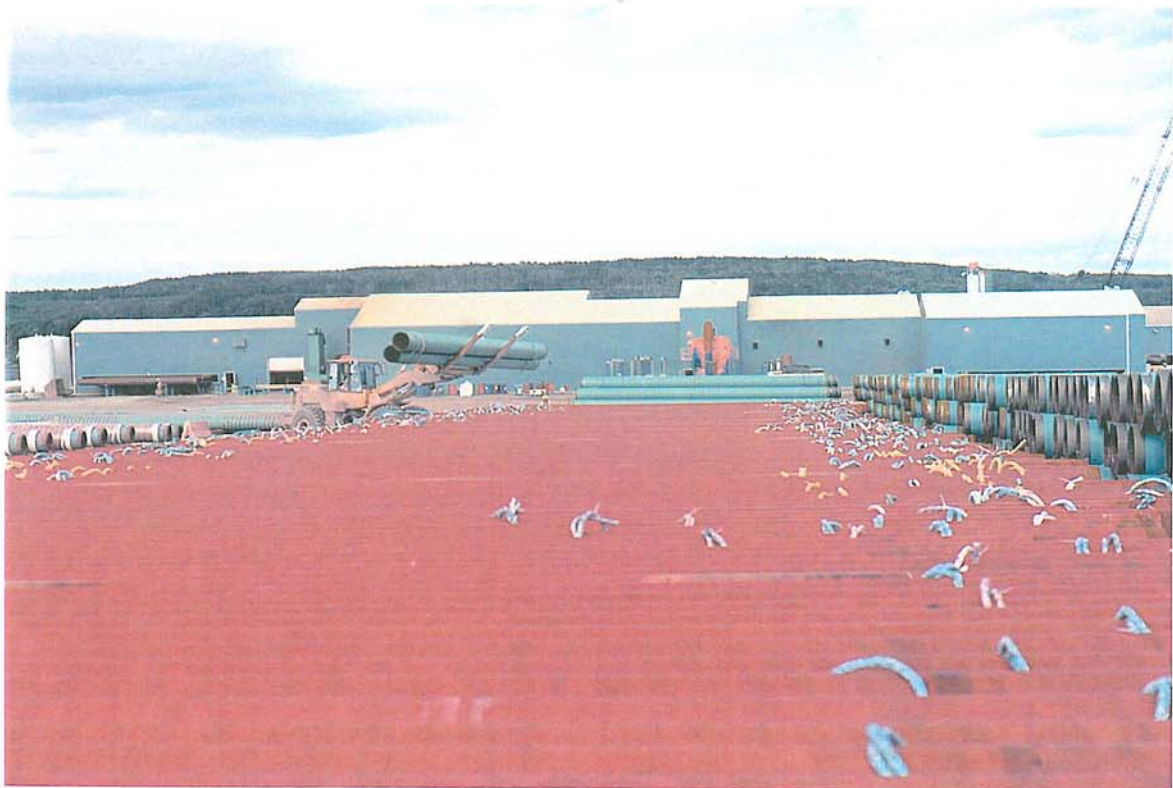
Pipe yard and coating plant, Shaw & Shaw, Sheet Harbbour, N.S.
