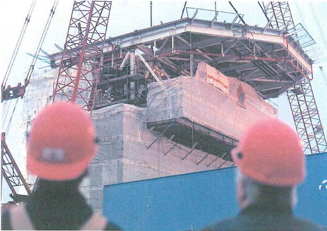
Placing helo deck on Living Quarters module. Fabco/CKT yard - Dartmouth.
