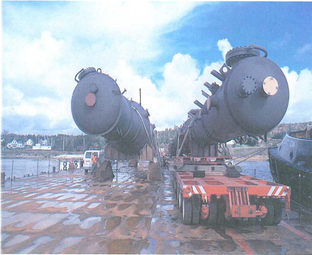
Deethanizer offloading at Goldboro Wharf.
