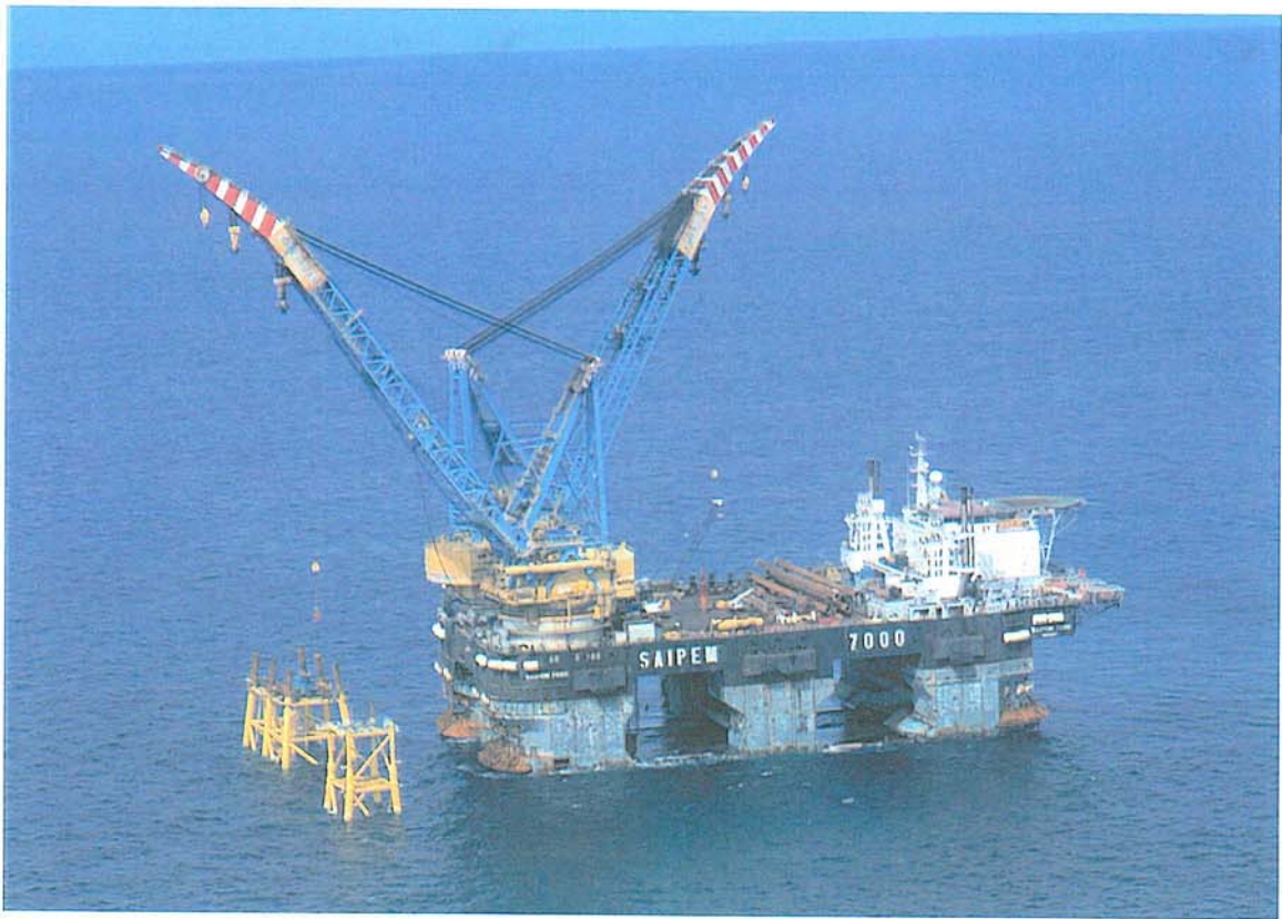
S7000 installing Thebaud jacket offshore.
