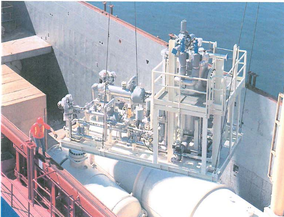
Loading produced water package and pressure vessels fabricated in Dartmouth for Teeside UK-Thebaud Process Deck components.
