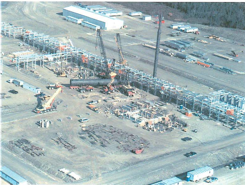
Deethanizer Tower and Pressure Vessels being installed at the Gas Plant in Goldboro.
