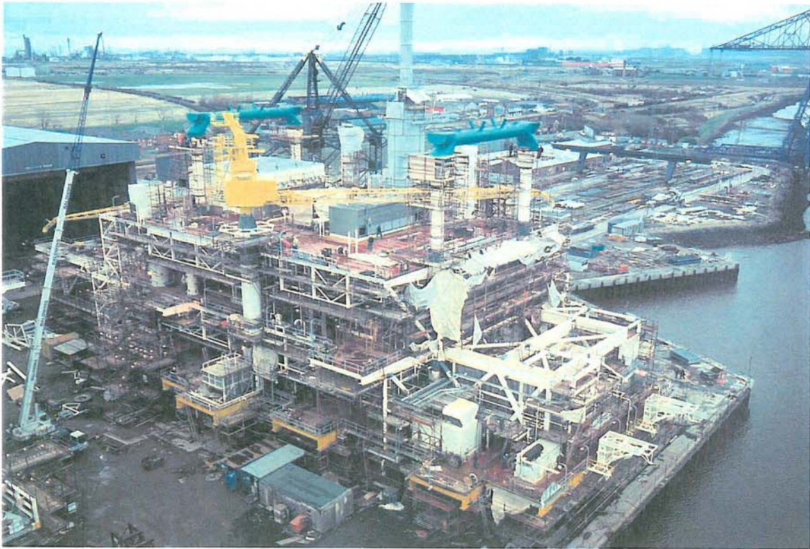
Thebaud Process Deck at Kvaerner, Teeside.
