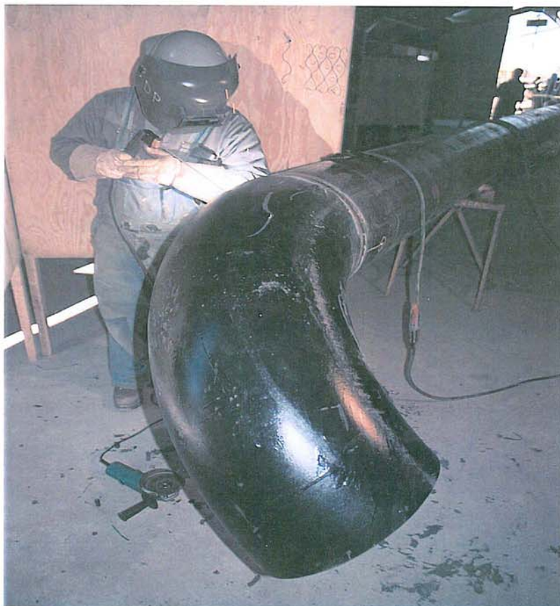
Pipe fabrication A.B. Mechanical - Louisdale, N.S.
