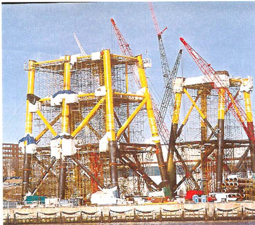
Early Jackets under Construction in Dartmouth Yard
