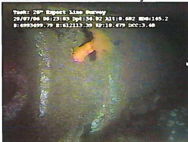
Figure 2-3 Sea anemone and shell debris near field joint # 861 on export pipeline
