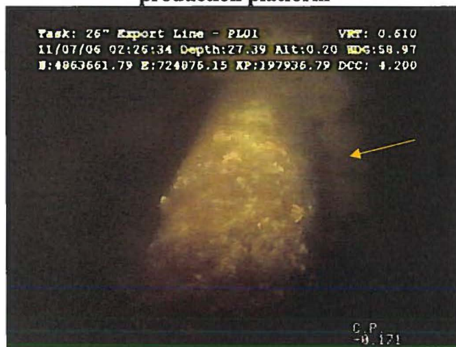
Figure 2-6 Export pipeline with associated protective mattress (arrow) near Thebaud production platform
