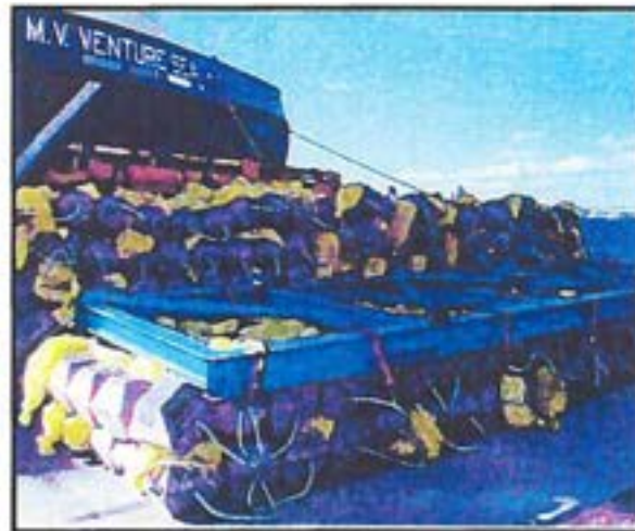
Photo 11 Anti-Scour Mattresses—Note Plastic ‘Seaweed’ Fronds
