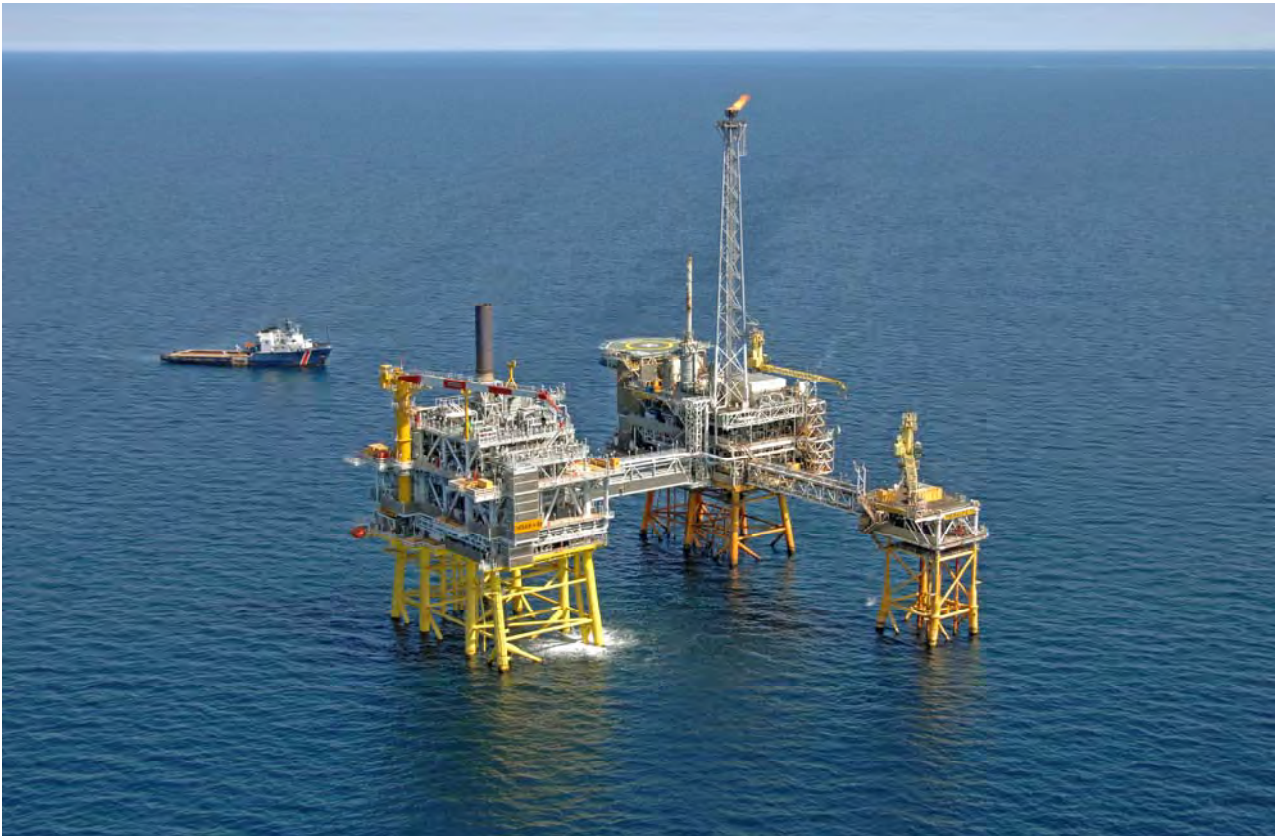
Thebaud Central Processing Facility – Offshore Nova Scotia
