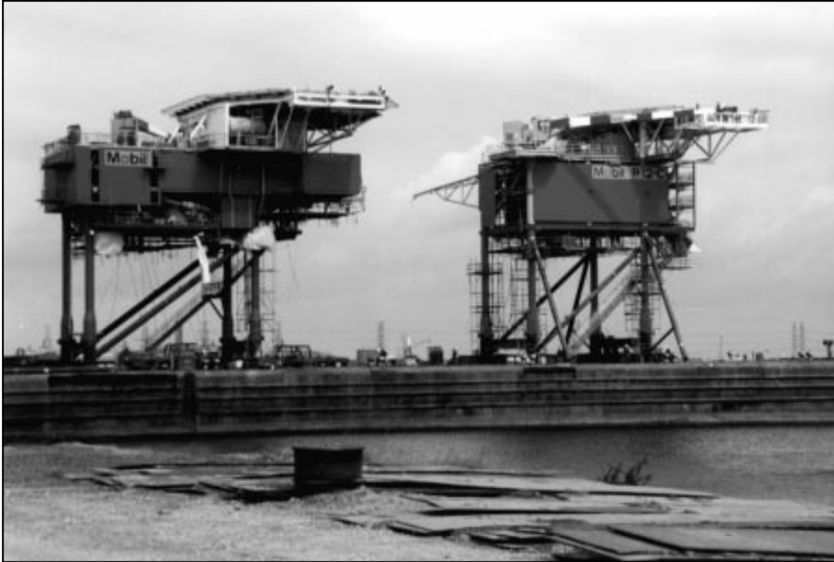
Figure 6.5.1: Example of Offshore Platforms
