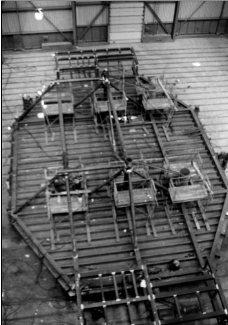
Figure 6.5.3: Module Deck Construction
