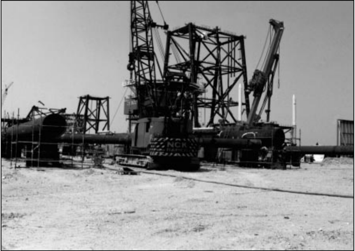
Figure 6.5.2: Jacket Erection
