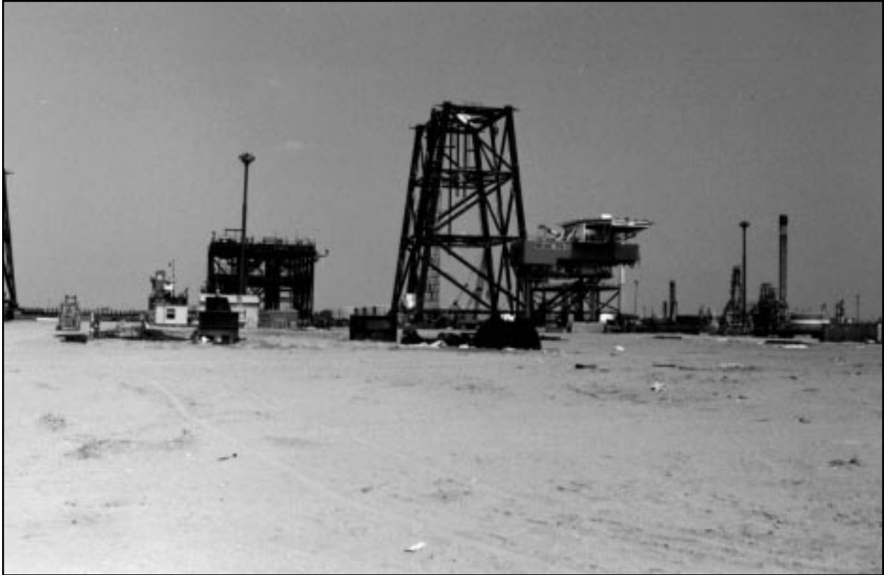
Figure 5.2.1.1: Typical Jacket Structure
