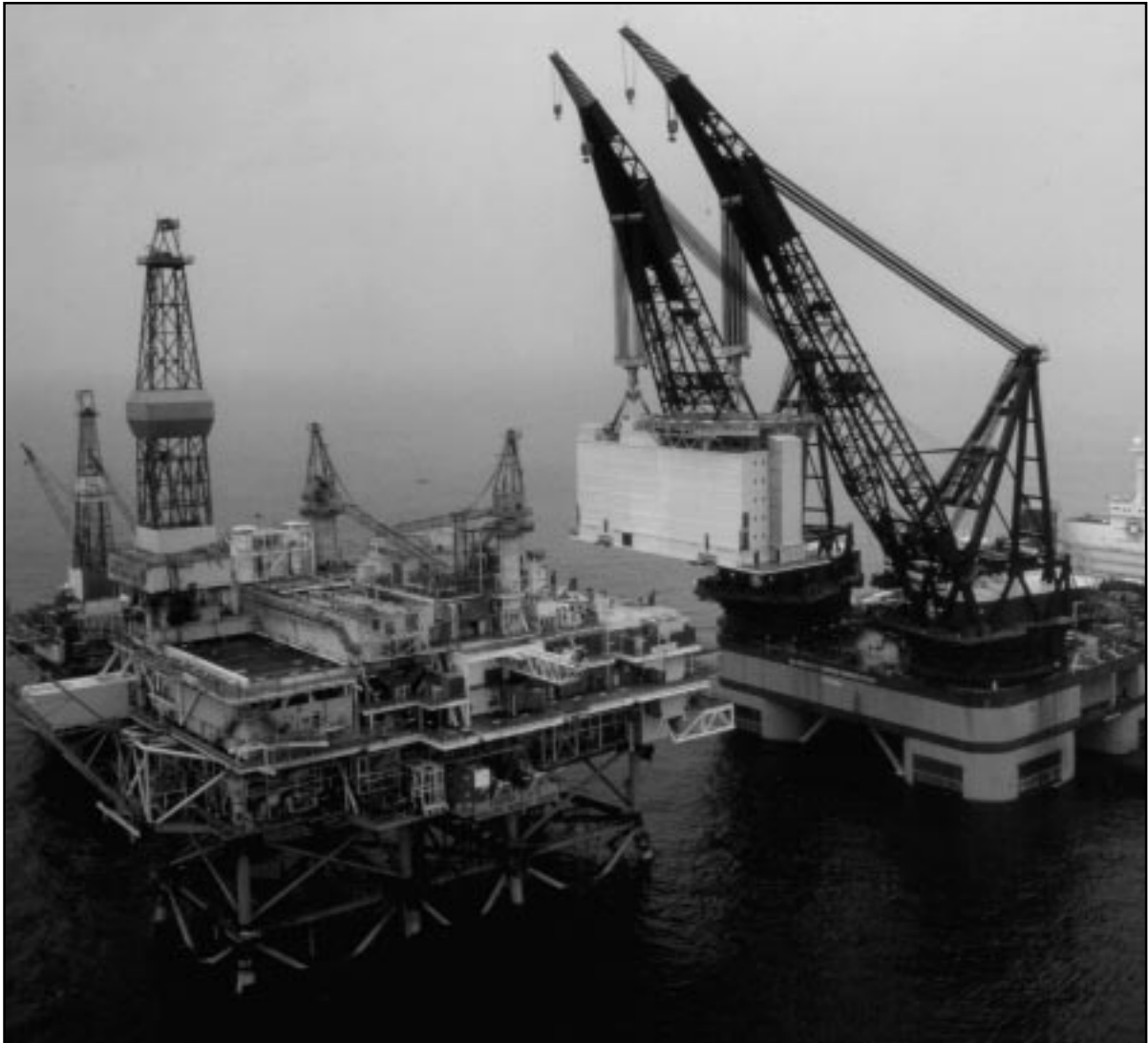
Figure 6.5.4: Heavy Lift Barge Installing Living Quarters
