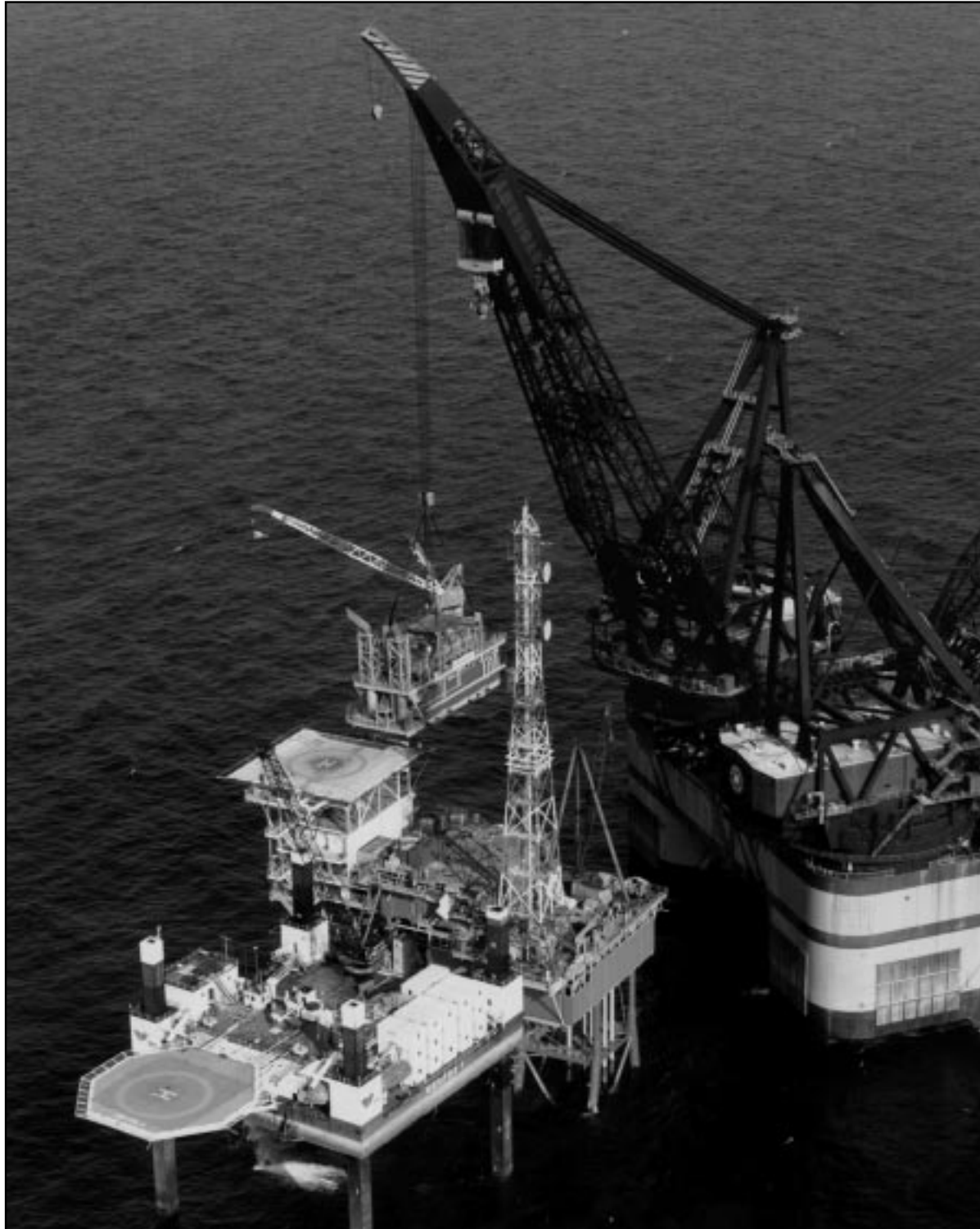
Figure 6.0.1: A Heavy Lift Vessel Installing a Compressor Module At An Offshore Platform. In the foreground is a construction support jack-up.
