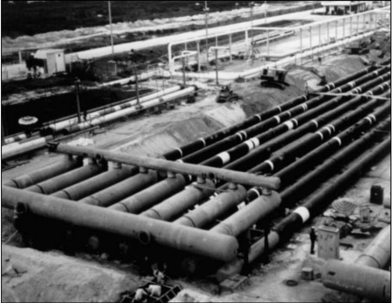
Figure 5.3.2.1: Typical Slugcatcher
