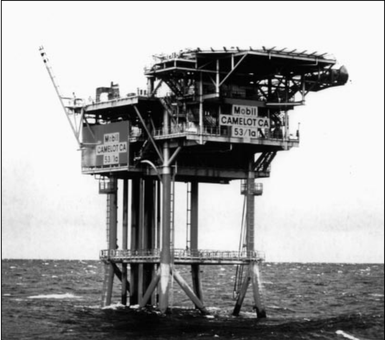
Figure 5.2.3.1: Typical Satellite Platform
