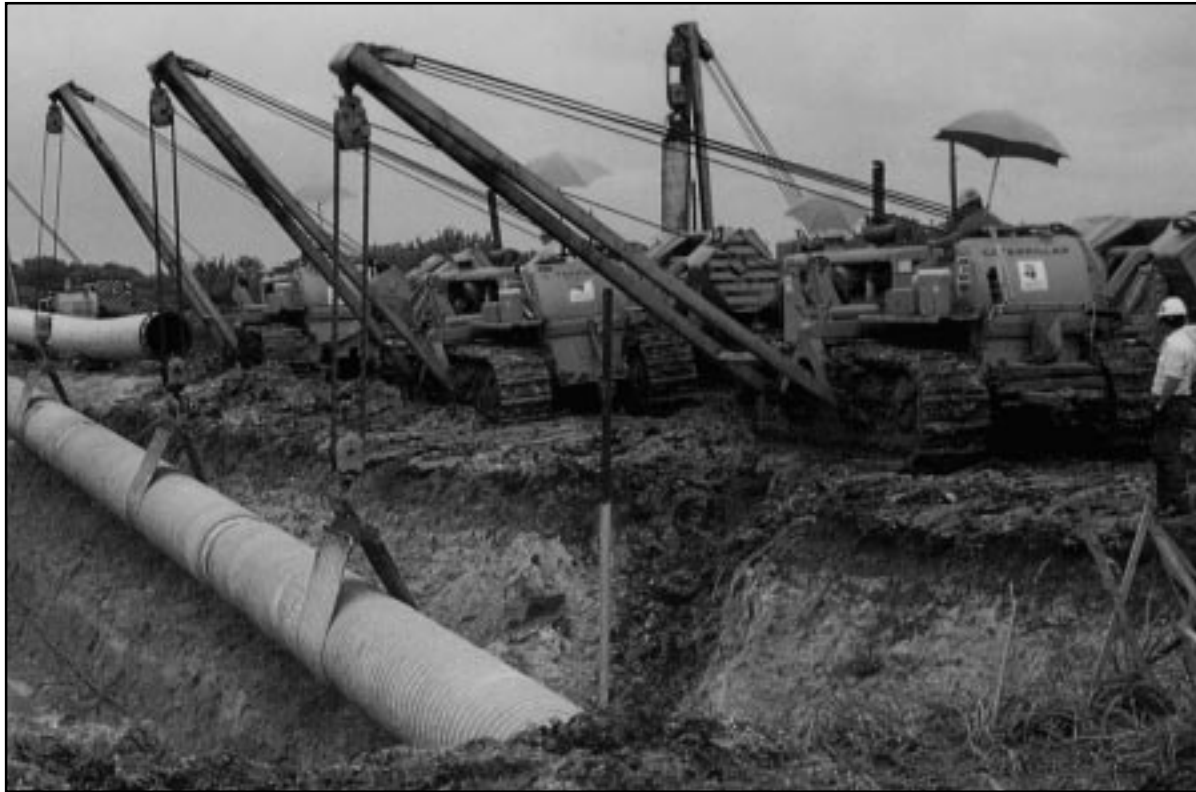
Figure 6.5.6: Onshore Pipeline Construction Spread
