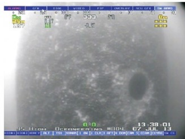
Dense mussel patches near the top of the leg, with some possible Metridium senile .
