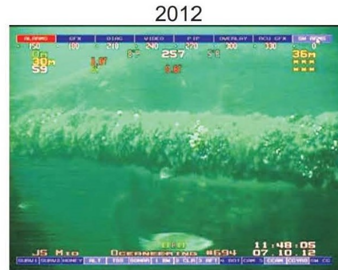
Significant growth of marine fauna on East horizontal bracket at WHPS M-79A in 2012.
