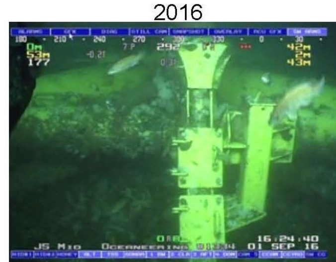
Minimal marine growth at MG-14 between Legs 2 and 3 which were cleaned in August 2016. Cunner are present.
