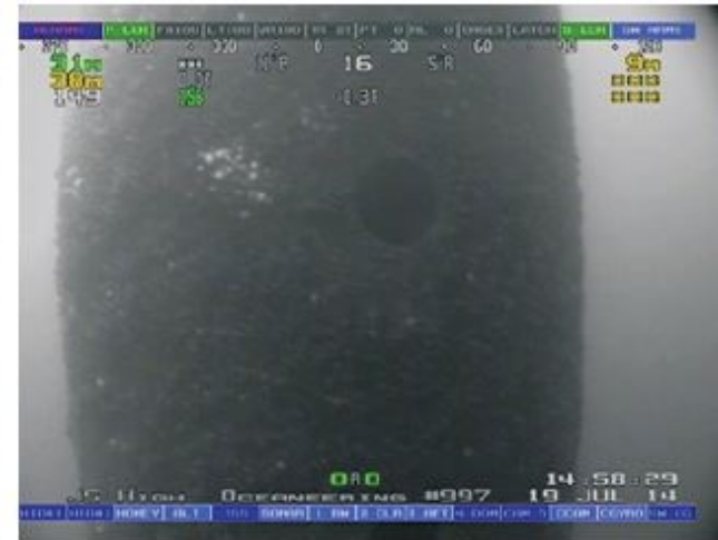
Increased mussel coverage (almost 100%) near the top of the leg with some possible Metridium senile .
