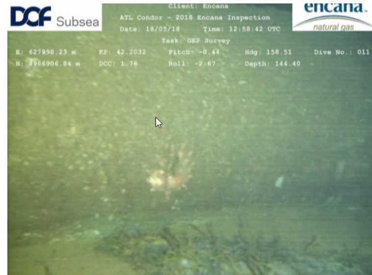
Soft debris (netting) at KP 42.203
