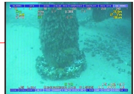
Dense hydroids, and sea star at the base of Leg 2.
