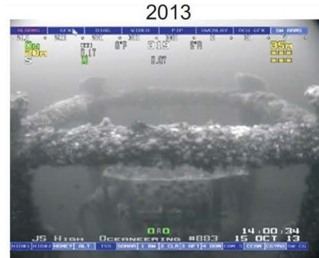
Significant growth, and 100% coverage of marine fauna on the East horizontal bracket at WHPS M-79A in 2013.
