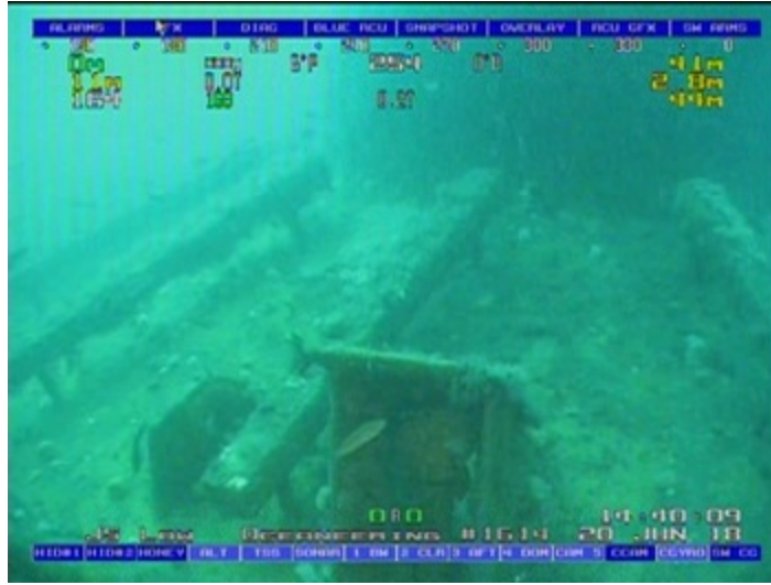
Base of PFC Leg 2 with minimal marine growth and cunner swimming around base
