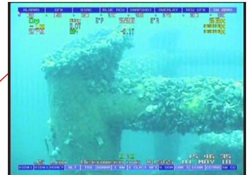
Marine growth is starting to recolonize at the top of Leg 3 where it was cleaned in 2017.
