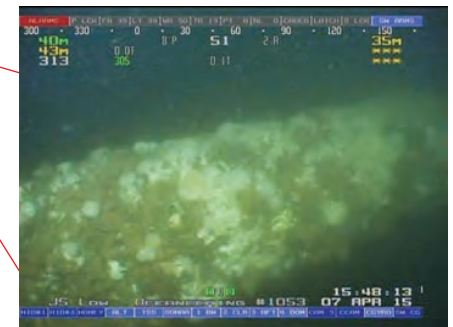
South horizontal bracket with frilled anemone and sea star on top of blue mussel.
