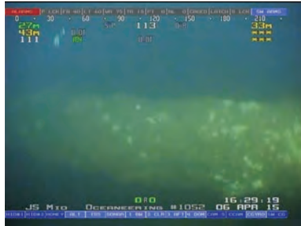
Dense mussel with hydroids and frilled anemone on the north crossbar between Legs 1 and 2.
