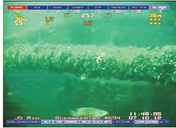
Significant growth of marine fauna on East horizontal bracket at WHPS M-79A in 2012.
