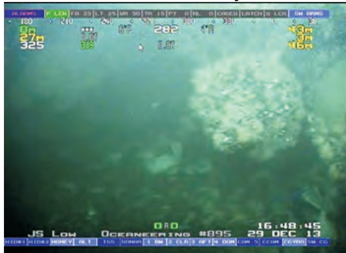
100% coverage of future flange cap. Increased blue mussel colonization with hydroids interspersed, in the 2013 survey.
