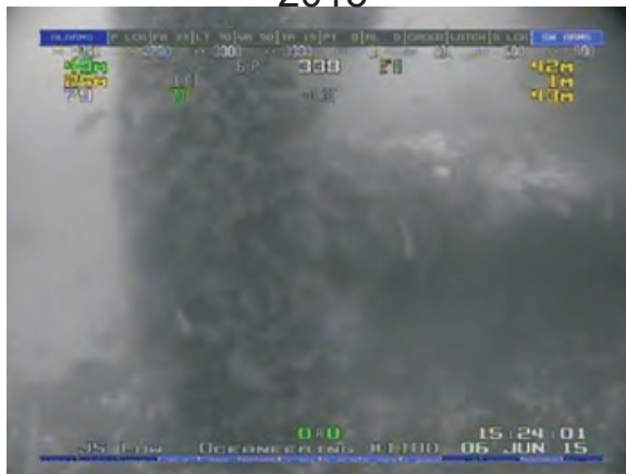
Dense blue mussel and hydroid coverage (100%), with patches of frilled anemone in the 2015 survey at the base of Leg 4.
