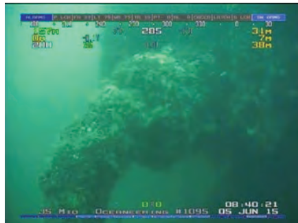
Dense mussel coverage with sea stars and hydroids on the subsea tree / flowline.
