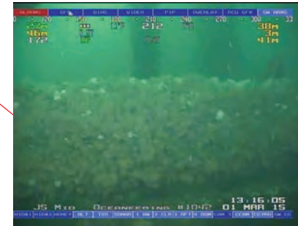
Dense mussel with hydroids over top, interspersed with frilled anemone on the lower crossbar off of Leg 3.
