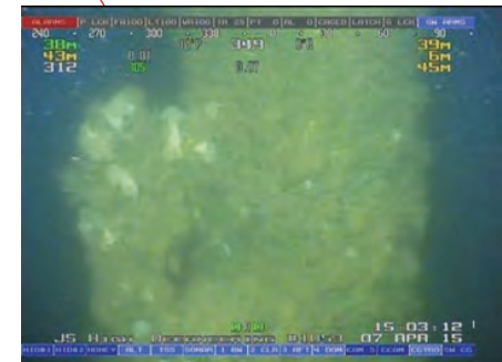
Dense mussel with hydroids over top, and some frilled anemone on Anode 6, mid-way up Leg 2.
