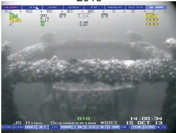
Significant growth, and 100% coverage of marine fauna on the East horizontal bracket at WHPS M-79A in 2013.
