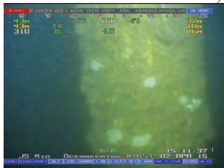
Hydroids and some frilled anemones on the lower part of Leg 4.
