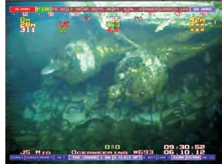
Increased coverage of future flange caps R-8 and R-9 by hydroids in the 2012 survey.
