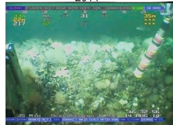
100% coverage of marine fauna on the East horizontal bracket at WHPS M-79A in 2014. Appears to have changed little since the 2013 survey.
