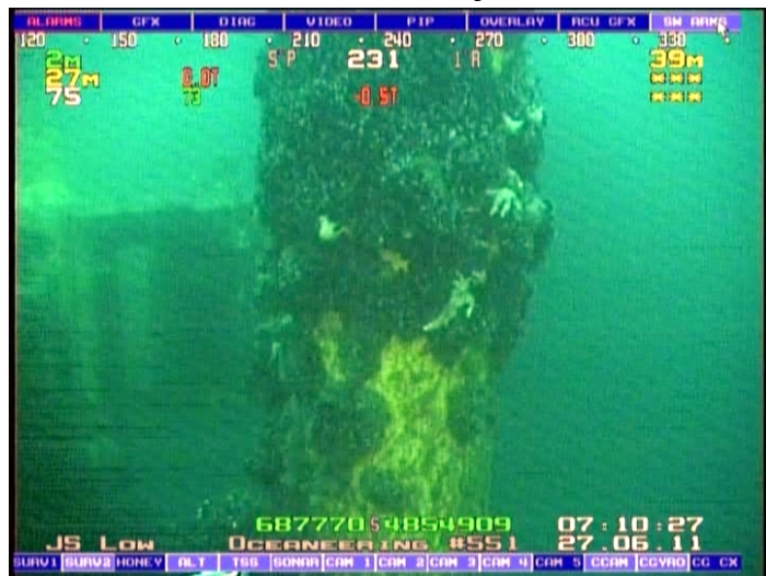
Blue mussel growth starting at 4 metres above the seafloor on Leg 2 at WHPS F-70 in 2011 survey
