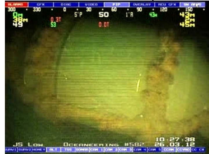
Significantly greater colonization of Tubularian hydroids on straps of insulation cover M-79A flowline in 2012
