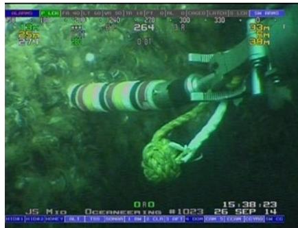
Dense mussel and hydroid coverage on the lower crossbar between Legs 2 and 3
