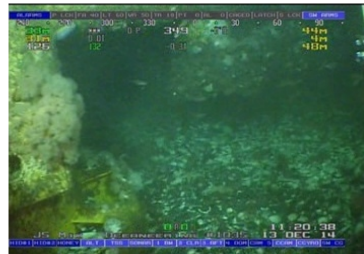
Dense mussel coverage on anode An04. Increased numbers of frilled anemones in the 2014 survey, as opposed to sea cucumbers in 2013.
