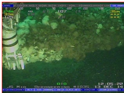
Dense hydroids and frilled anemone on the west horizontal brace between Legs 1 and 4
