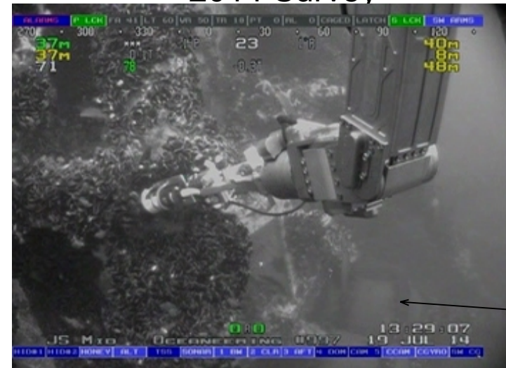
Growth appears similar to the 2013 insulation cover (only video/photo available of lower riser area from 2014 videos).
