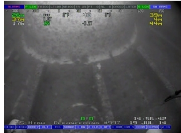
Less marine growth on the PFC leg in 2014 than 2013. This could be due to cleaning.
