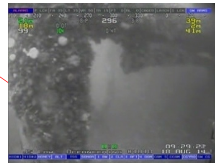
Dense blue mussels with some frilled anemones near the base of Leg 3, showing Anode 3
