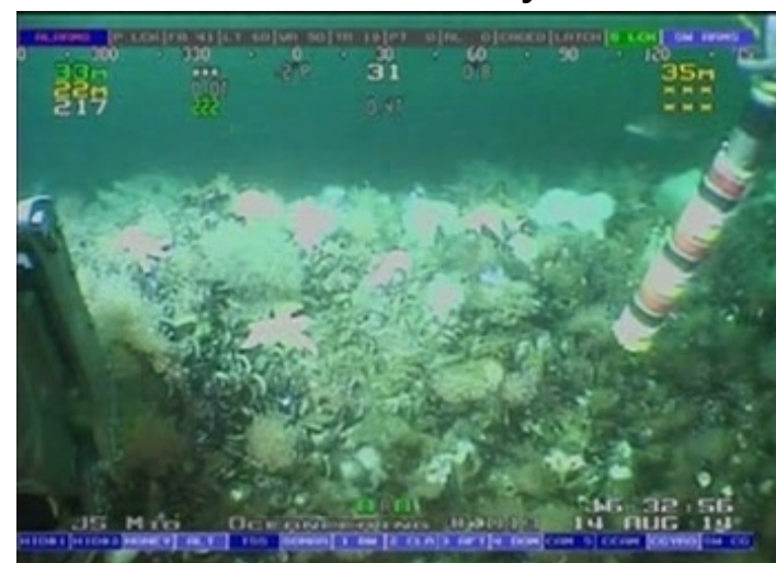
100% coverage of marine fauna on the East Horizontal Bracket at WHPS M-79A in 2014. Appears to be little change from the 2013 survey.
