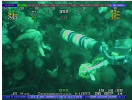
Dense coverage of mussels, hydroids and seastars on the south crossbar between Legs 3 and 4
