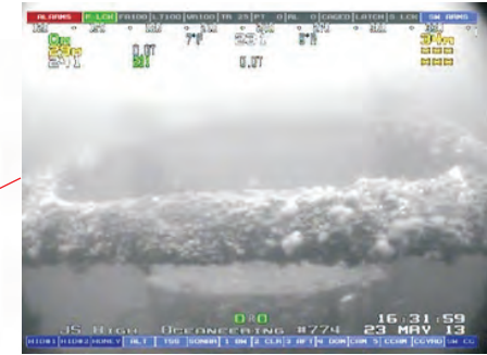
Abundant blue mussel growth with hydroids on the East horizontal bracket
