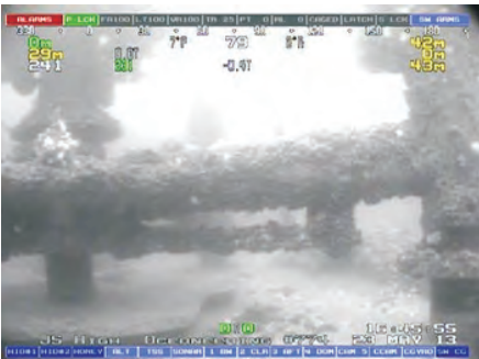
Blue mussel colonizing anode AN04
