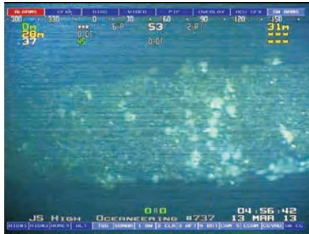
West horizontal bracket densely colonized by blue mussels with sea stars and anemone.
