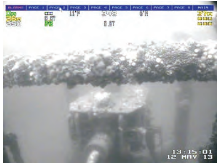
A horizontal brace with dense patches of blue mussel, hydroids and sea anemones
