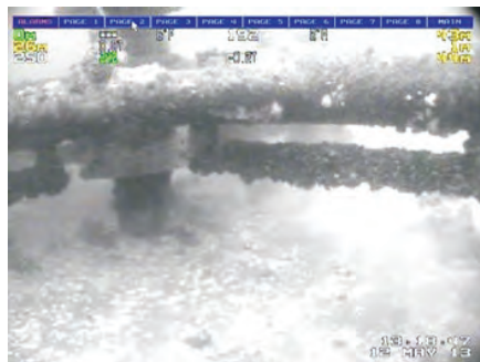
Dense blue mussel coverage on an anode
