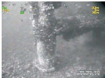
Dense coverage of blue mussel with some sea anemones at the base of Leg 4
