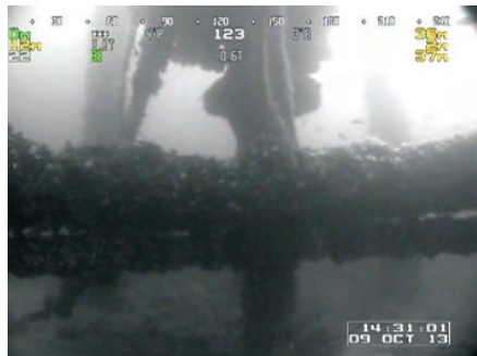
Dense blue mussel coverage on the inside of the WHPS
