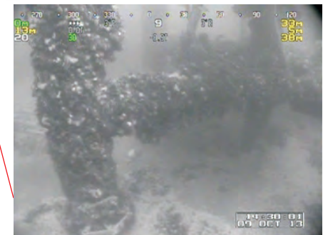
Blue mussel and sea anemone coverage at the base of Leg 2, HB01-2 and AN02
