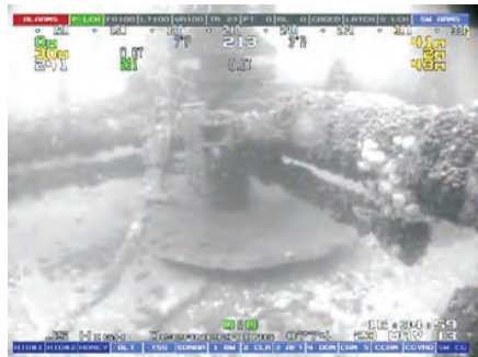
Blue mussel and sea anemones near the base of the Subsea Tree
