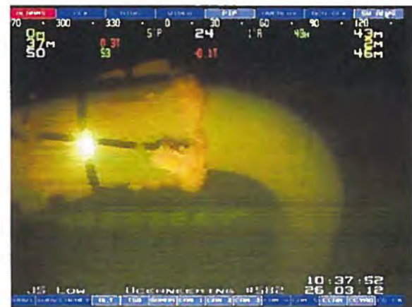
Colonization of Tubularian hydroids on VIV suppression strakes of D-41 in 2012 survey - Note the area colonized in 2012 does not have any straps in the general area in 2011
