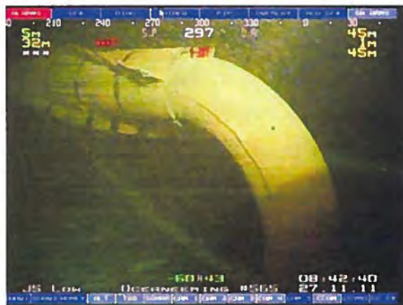
Absence of Tubularian hydroids on VIV suppression strakes of D-41 in 2011 survey
